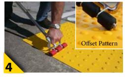
To insure a secure bond is achieved, roll the mat both lengthwise, widthwise and most importantly along the edges, with the handheld *RediMat™ Roller. For mats with an offset pattern,* hold the roller at a 45° angle and use the outer roller pad to roll between the domes diagonally from front to rear and along the edges.
