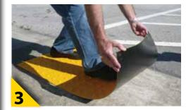
Roll and press the exposed portion onto the surface. While standing on the attached end, peel the remaining sections of the backing and press and roll onto the surface.
