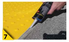
Cut the nozzle of the sealant tube at the 1/4 in. mark. Apply a smooth, thin bead of sealer around the perimeter (sealer is not required between adjoining mats). Mats are ready for immediate use once installation is completed and edge sealant has dried to the touch. *Tip: To make the edge sealer dry faster, mist with plain water.*
