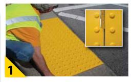
After ensuring "General Conditions" (refer to box on left) have been met, and surface has been properly cleaned, place mat(s) in desired final position. *If mats are placed side by side, leave a 1/8 in. gap between them.*
