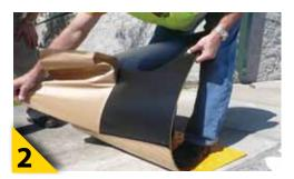
While standing on the mat to prevent movement, remove one section of the paper backing.
