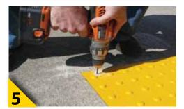
Using the drill and a 5/32 in. masonry bit, drill through the pre-drilled holes into the concrete to a depth of 1 1/4 in. If the mats are trimmed so a pre-drilled hole is removed, a new hole must be drilled in the mat using a 3/8 in. standard drill bit, 2 in. from the side edge and 1 in. from the beveled edge.
