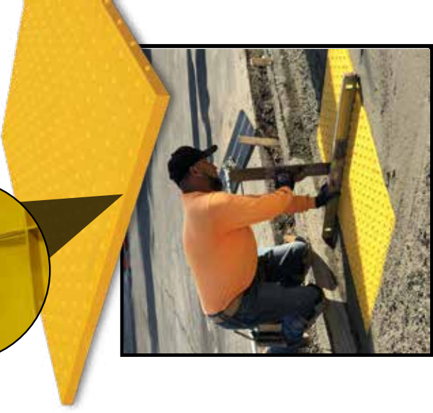
Pre-drilled holes for solid embedment.
